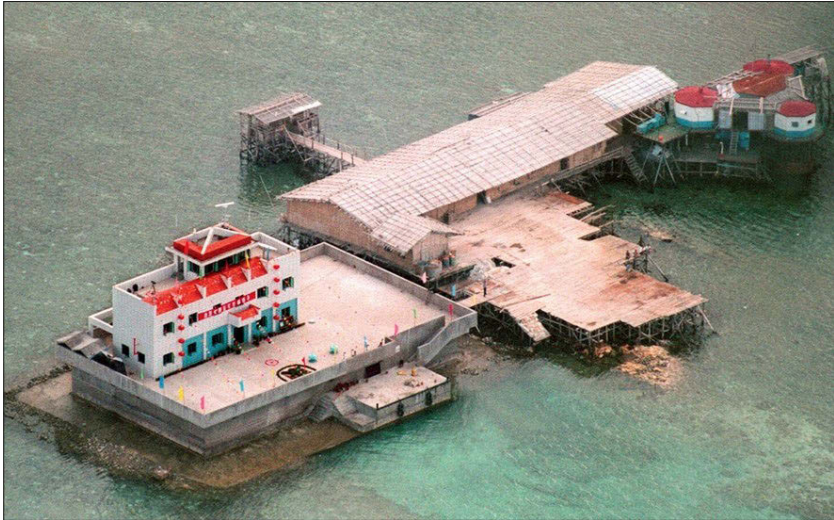
Figure 30: Aerial Photograph of Structure on Mischief Reef Supplemental Written Submission, Vol. II, p. 126.
