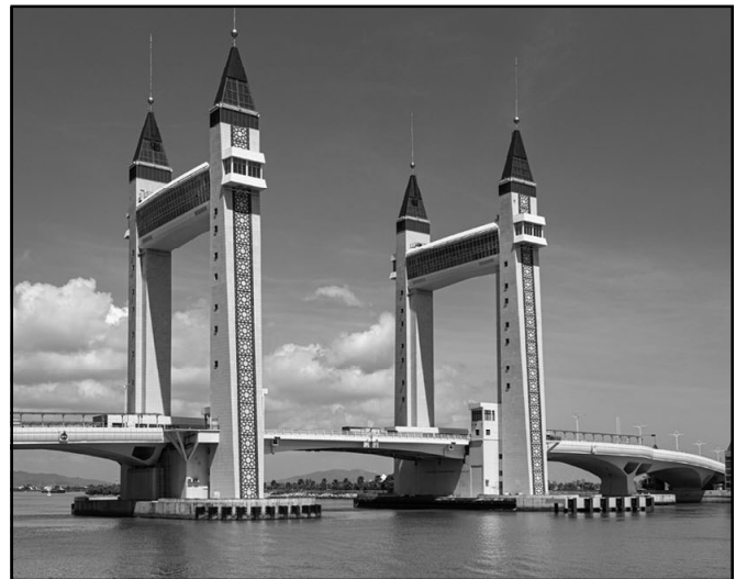
Kuala Terengganu drawbridge
